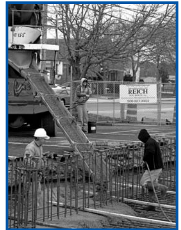
Above: pouring footings Left: pouring the foundation wall Middle: erecting the frame Right: installing walls Bottom Left: finishing the concrete floor Bottom Right: installing Extech® façade
